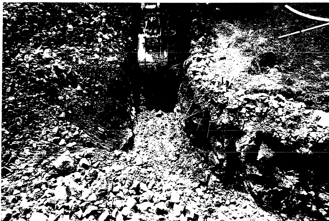
No. 2: Solid rock trench walls. Broken up with backhoe pounding.
