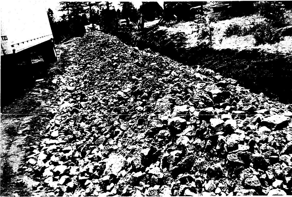
No. 3: Broken basalt rock, no clean backfill present.
