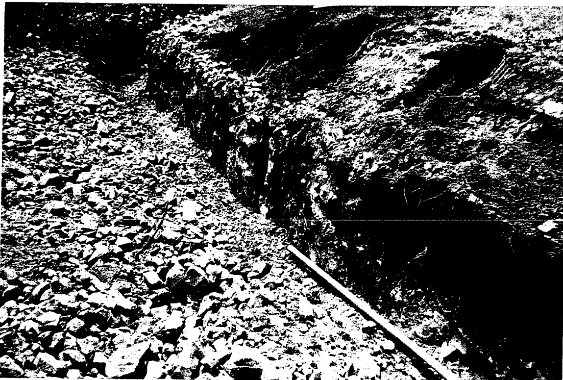
No. 1: Solid rock. Little or no backfill present. Sifting required.
